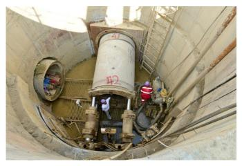
The Project is divided into six packages, the works of two of them -Packages 4 and 5were awarded from DJB to the Joint Venture formed by the companies DS Construction, Fegshun and Wabag. In order to complete part of the pipe jacking works of the Package 4, the JV acquired from TERRATEC a DN1600 Microtunnelling System composed of a Slurry MTBM, Slurry Transport System, Main Jacking Station, Intermediate Jacking Stations, Lubrication System and Separation Tank.
